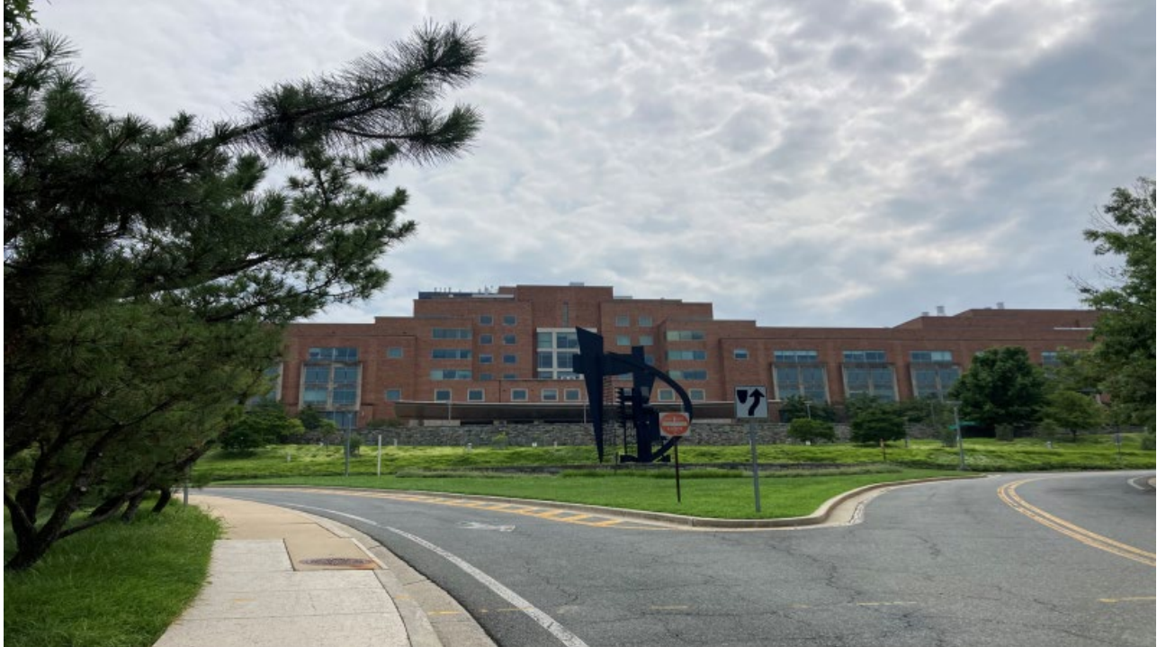
View of Building #10 from the front entrance
