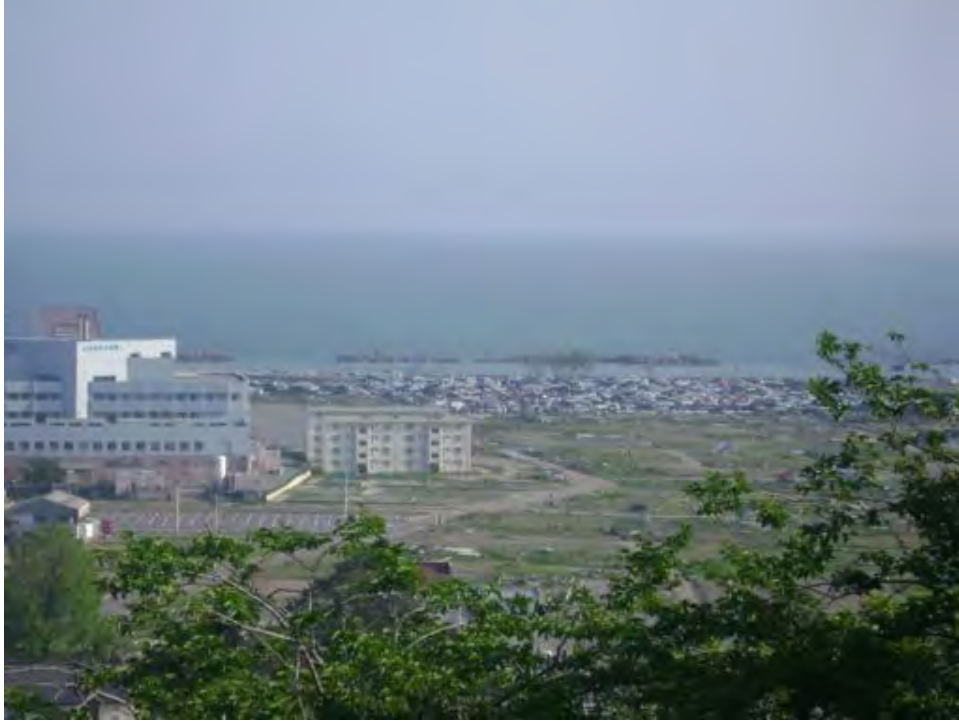
A destroyed hospital to the left and destroyed cars to the right.
