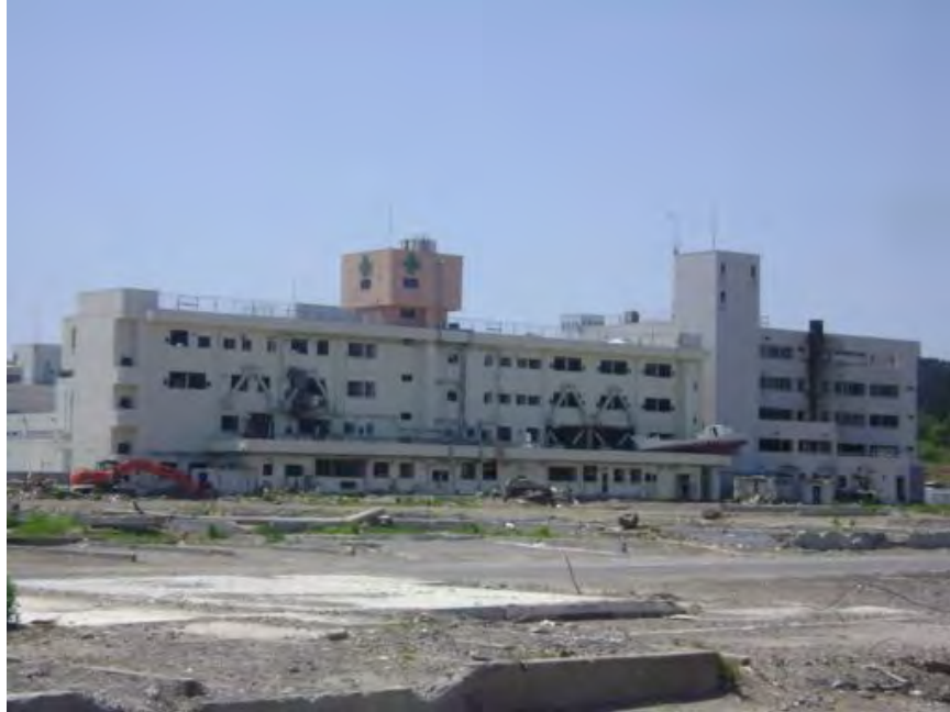
Shizugawa Hospital - May 2012 Note the boat resting on the second floor
