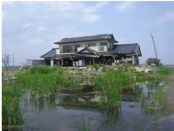
Hollowed out, destroyed homes
